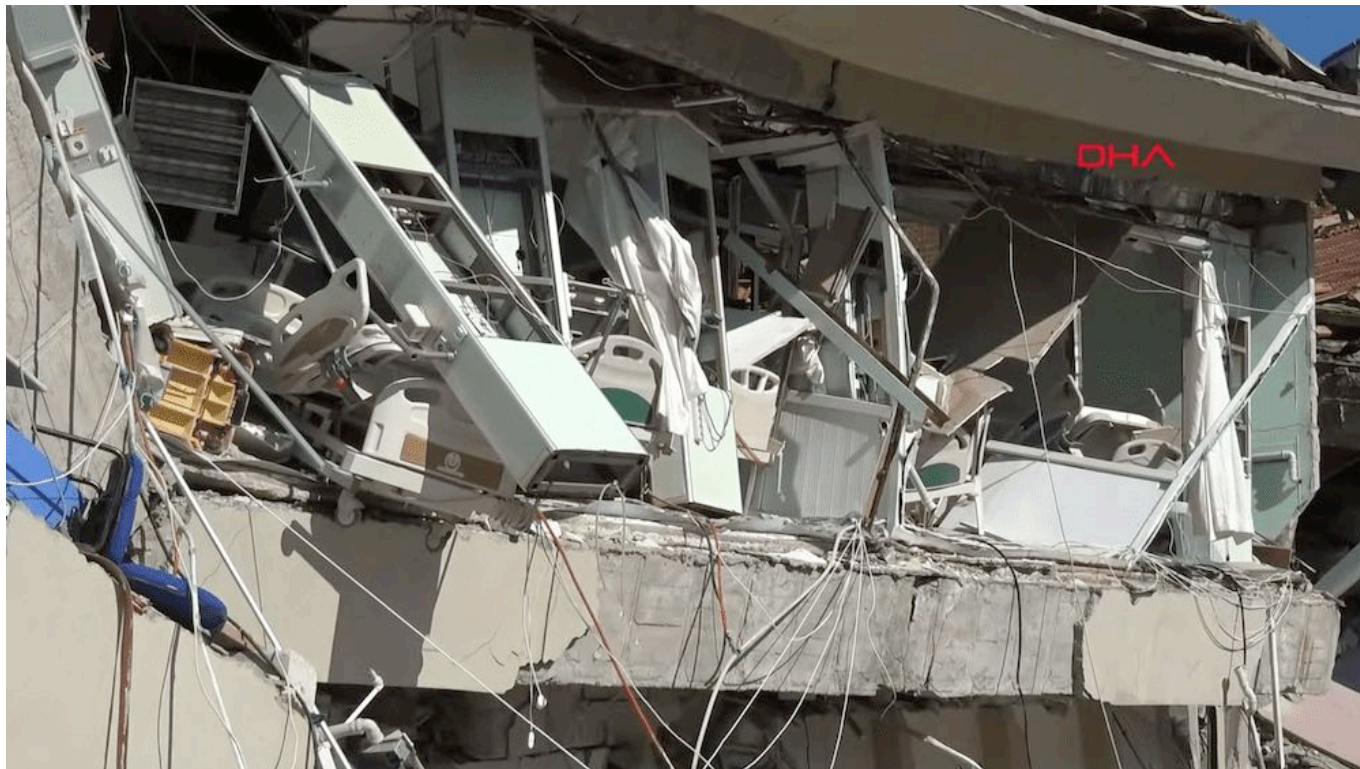
Hospital beds tip over the edge in part of the Hatay Education and Research Hospital in Antakya, which collapsed in the earthquake.
