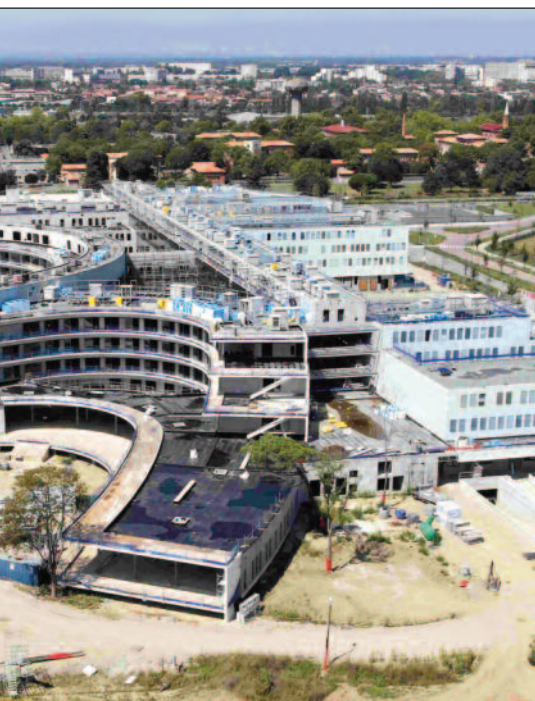
Like a phoenix from the ashes. The Toulouse oncopole is built on land left devastated by a catastrophic explosion at a chemical works in 2001. The University Cancer Hospital – the curved building in the centre – will open in early 2013
